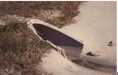
Use **Beveling of Pipe End** (719-610-00) when specified
